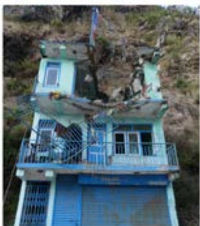
Damage caused by landslides in Sindhupalchok District, Nepal. Credit: © N. Rosser, 2016. Reproduced with permission.
